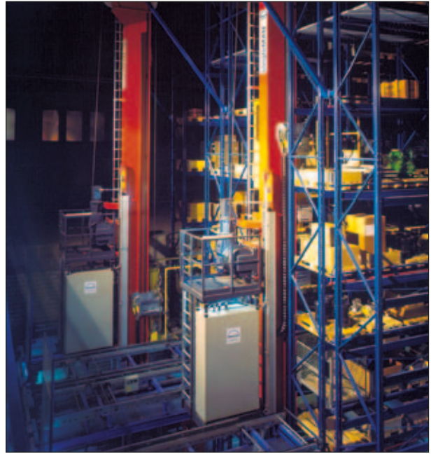
MAN Logistics: Hochregallager
